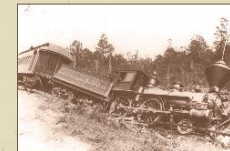
Train derailed from tracks by a four-foot high wall of water when the Charleston earthquake burst the mill dam at Langley Pond near Aiken, SC.
